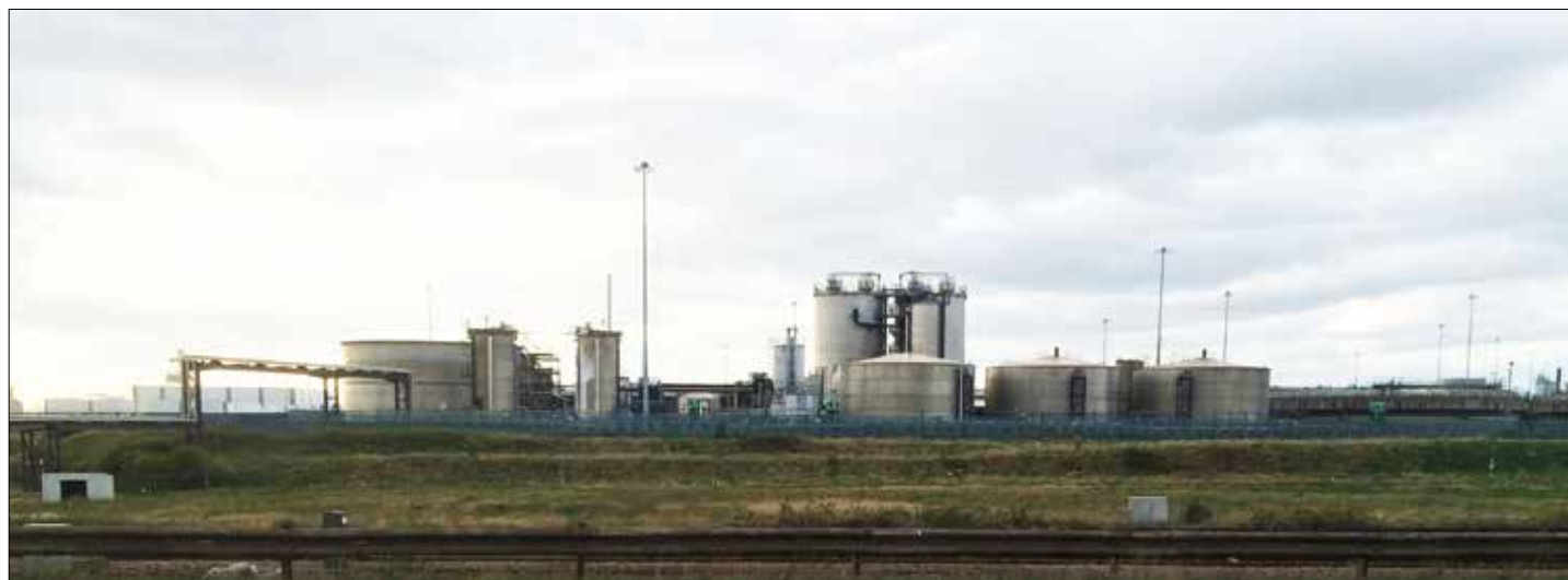
NWL Brand Sands WWTW
