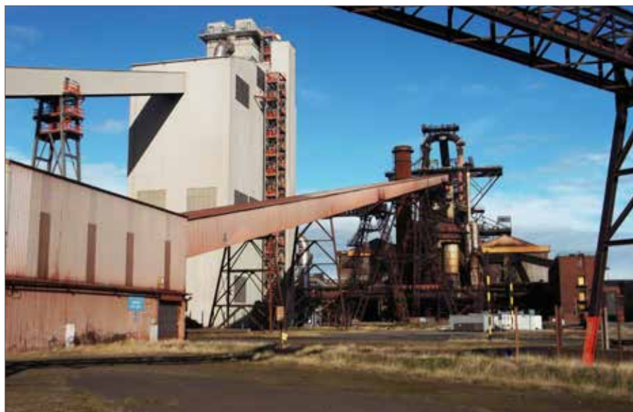
Pulverised Coal Injection Plant at Redcar Blast Furnace
