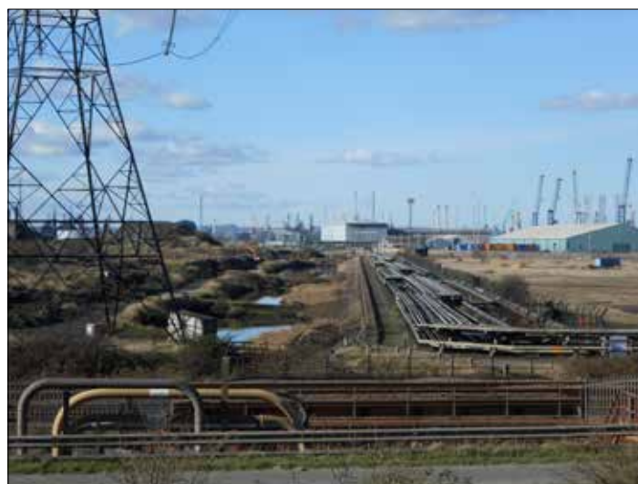
Sembcorp Corridor - West - to No.1 Tunnel
