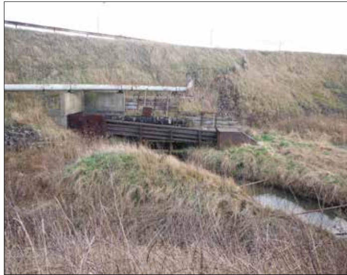
The Fleet - Culvert No.2
