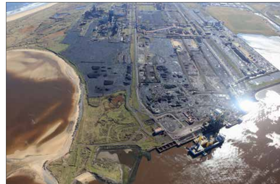
Redcar Bulk Terminal
