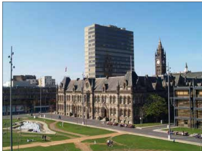
Middlesbrough Centre Square
