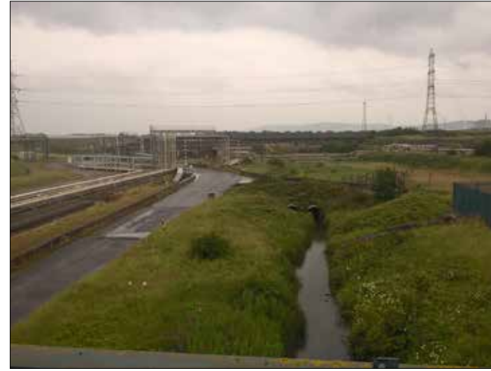
Sembcorp Corridor and Dabholme Gut south of WWTW
