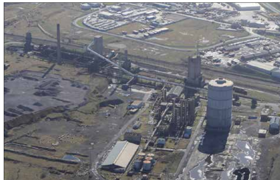
South Bank Coke Ovens
