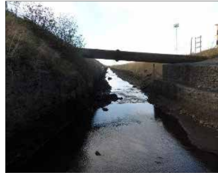
Lackenby Channel drainage cut
